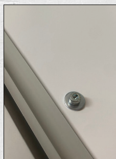
The 'hanging hooks' consist of Allen screws, washers, and nuts that fit perfectly into the premilled holes.
